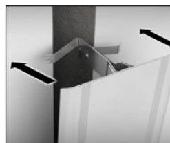
3. Push firmly into joint
