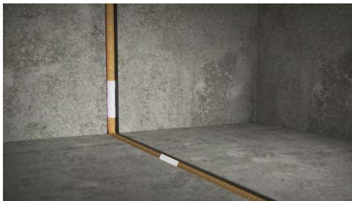
Application on floor and wall with junctions.
