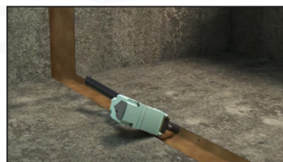
Fix the wings of the blanket to the slab every 20cm using a pneumatic nailer.
