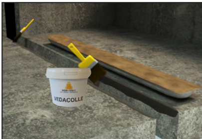
Apply the VEDACOLLE ® adhesive on 150mm depth on both sides of the joint.
