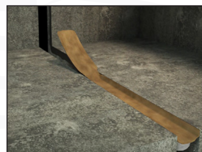
Insert the VEDAFEU M ® blanket into the joint.
