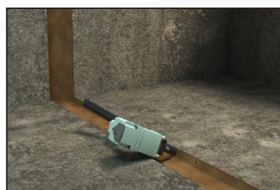
Fix the wings of the blanket to the slab every 20 cm using a pneumatic nailer.
