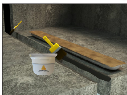
Apply the VEDACOLLE ®** adhesive on 150 mm depth on both sides of the joint.
