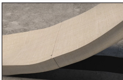
Handle with care to avoid damage to the junction. Insert the spliced blanket into the joint.
