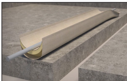
Preform the blanket in "U" shape, by folding it in its central part.
