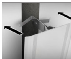
3. Push firmly into joint
