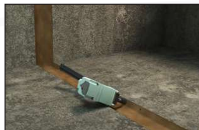
Fix the wings of the blanket to the slab every 20 cm using a pneumatic nailer.
