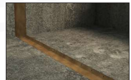
VEDAFEU M ® blanket after installation.
