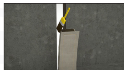
To splice two lengths of blanket, apply adhesive on the extremity of both blankets before compressing them together.
