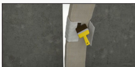
Put VEDAFEU linking material around the junction and seal it with some VEDACOLLE ® adhesive.
