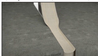
Insert the blanket VEDAFEU N20 ® into the joint before the adhesive dries.
