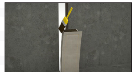
To splice two lengths of blanket, apply adhesive on the extremity of both blankets before compressing them together.
