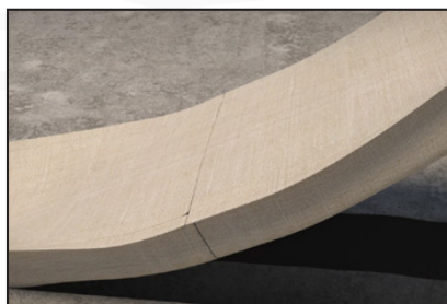
Handle with care to avoid damage to the junction. Insert the spliced blanket into the joint.
