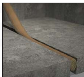
While the adhesive is still wet, insert VEDAFEU C ® by hands into the joint.
