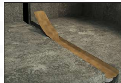
Insert the VEDAFEU M® blanket into the joint.
