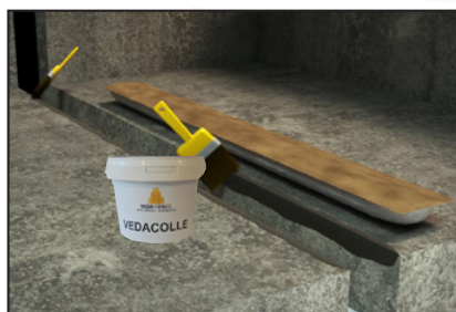
Apply the VEDACOLLE ®** adhesive on 150mm depth on both sides of the joint.
