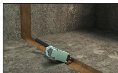
Fix the wings of the blanket to the slab every 20cm using a pneumatic nailer.
