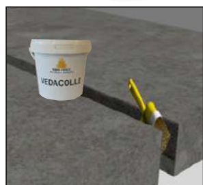
Apply a layer of VEDACOLLE®** adhesive with a brush on both sides of the joint.
